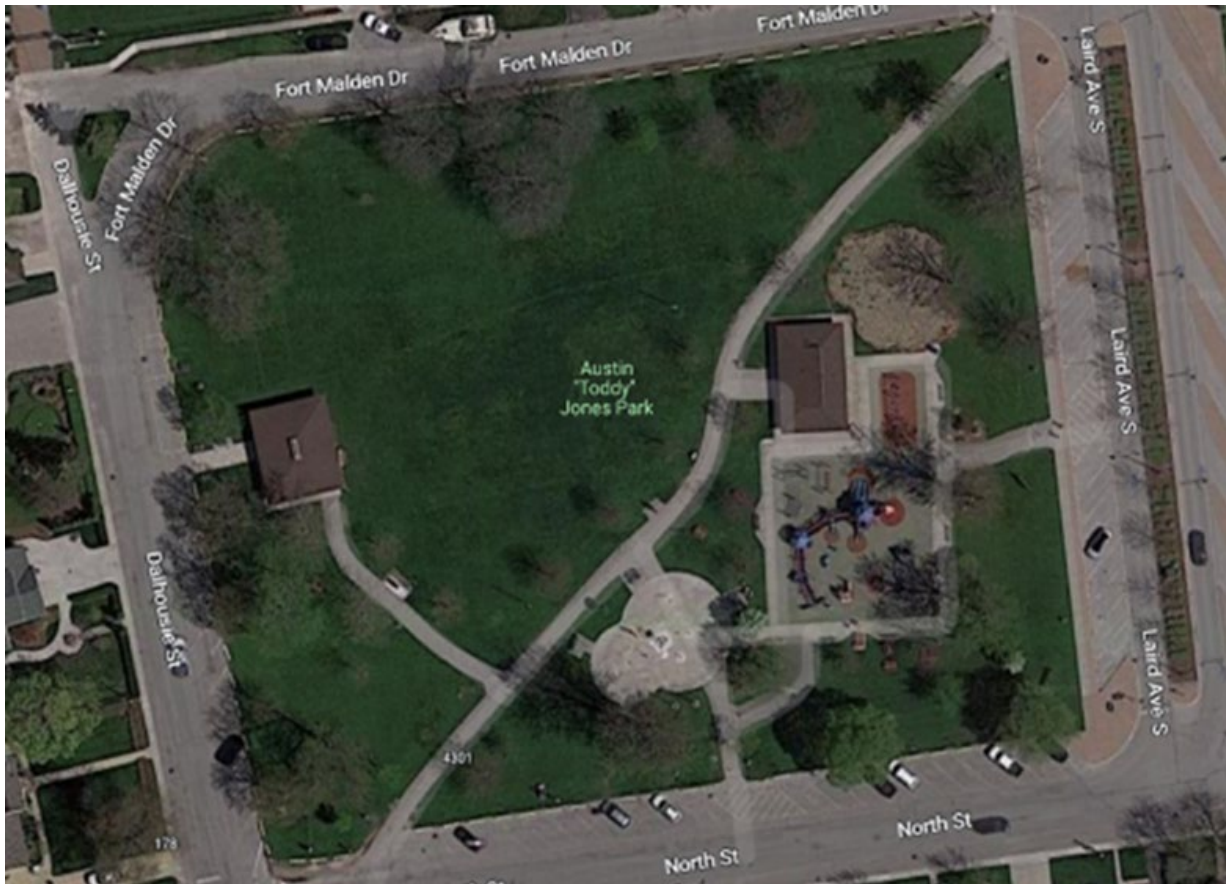
Figure 4-19: Austin “Toddy” Jones Park (the lack of AT facilities)
