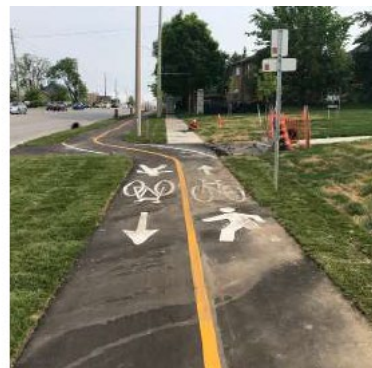
Multi-Use Path Separated by Grassy Boulevard, Richmond Hill
