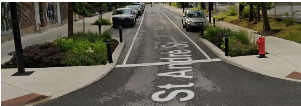
Figure 5-5: Curb Bump Outs on a street.
